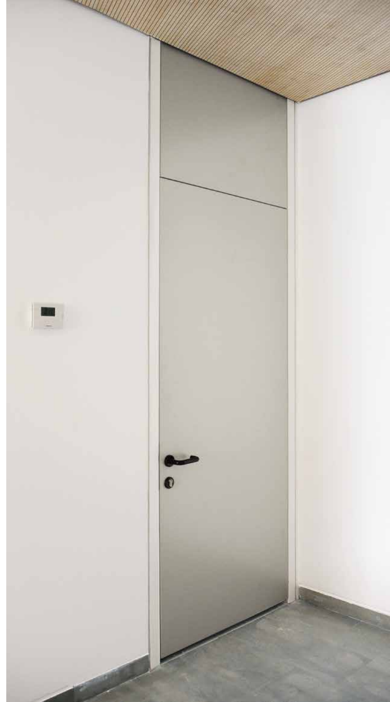
Dettaglio porta con sopraluce cieco a filo Detail of the door with with a blind overpanel transom
